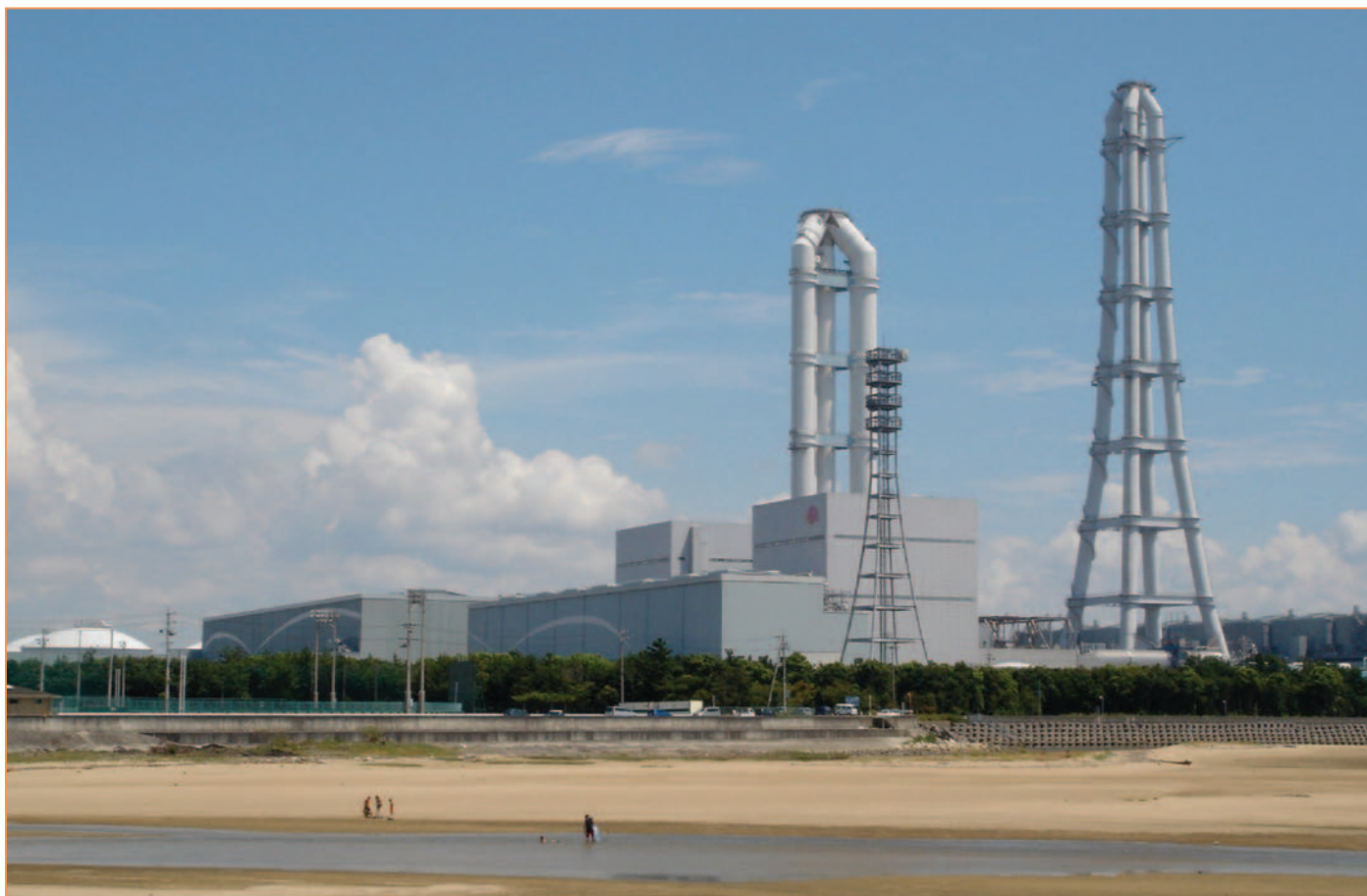
Kawagoe Thermal Power Station
